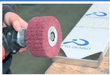
Finish of welds on a stainless steel sheet
